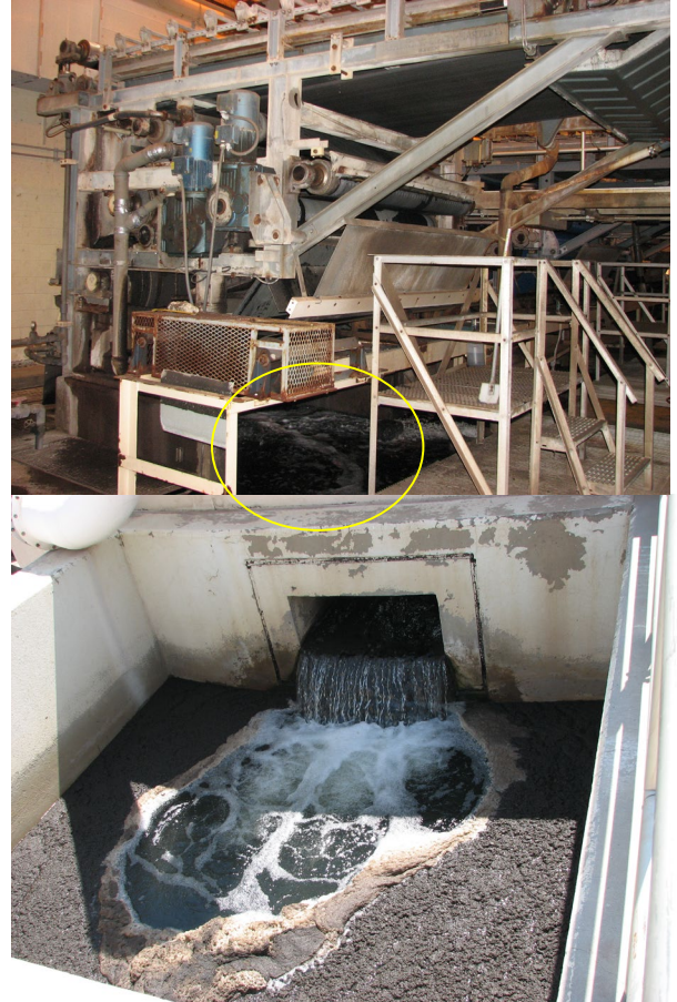
Belt Press Filtrate Wastewater
