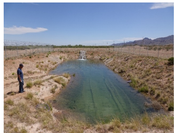
Figure 2. Infiltration Basin in El Paso, Texas
